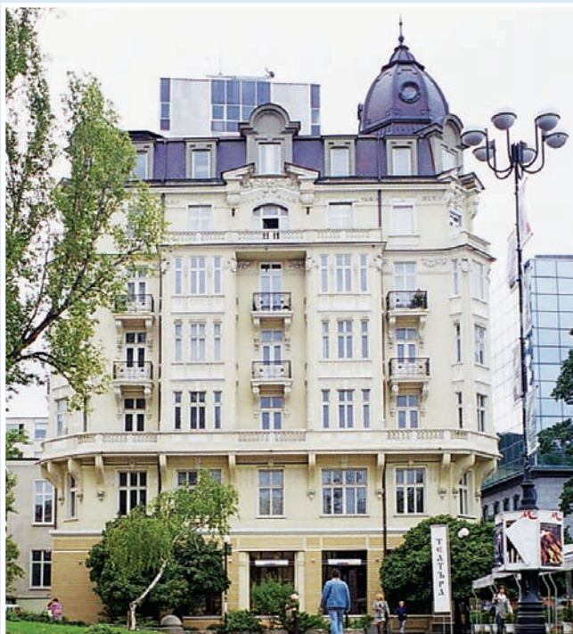
Reconstruction and restoration of the elevation of the building , used to be owned by Mr. Gendovitch, Sofia Employers: Gendovitch OOD and ING Bank The building is a cultural monument Total built-up area 1,200 m 2 August 1995 – January 1996 The majority of the sculptural elements have been restored, and 30 percent have been completely replaced.
